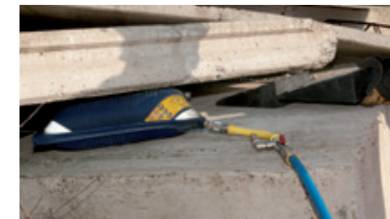
Lifting bag is inflated and backed up by stabilization blocks
